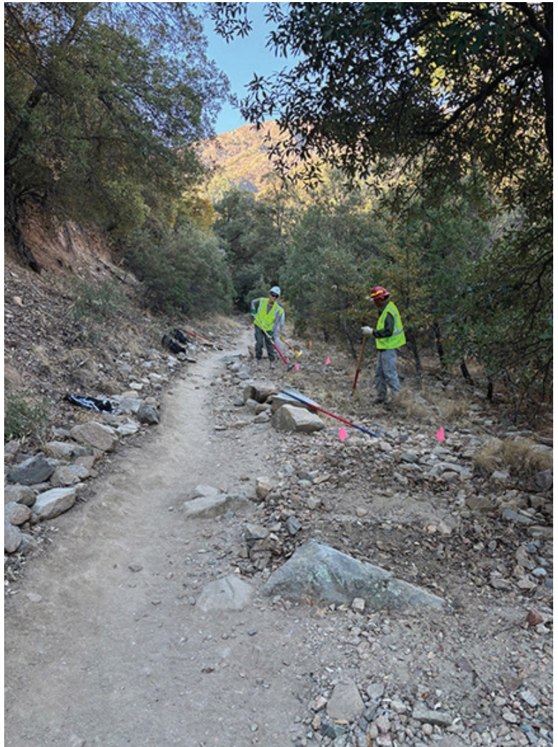
Stacey Barnes and David Linn work in the newly marked outsloped section while leaving the existing trail open to hikers.
